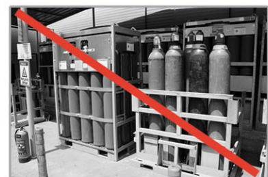
7/24 Own Nitrogen production (pic.1)
